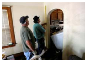
FEMA inspectors on site Credit: AP Photo/Seth Wenig
