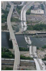
Interstate 35W Bridge Collapse Photo Credit: AP Photo/Star Tribune, David Denney
