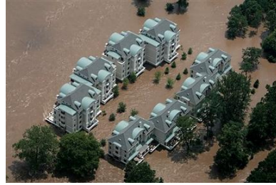
New Hope, PA condos flooded by the Delaware River.
